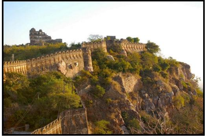
The Palace (Bikodan za Morganna el Oona) as seen from the Western Walls looking south. The zipline tower (Iejie Skar) is visible on the lower wall.
