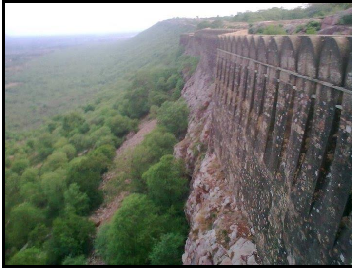
The Outer Walls are very high (60'-80')-(20'-40' Thick)
