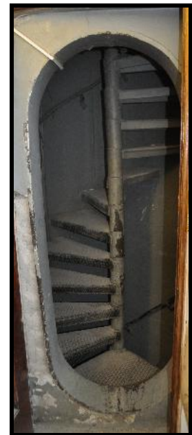
The Secret Stair shaft - 2A22
