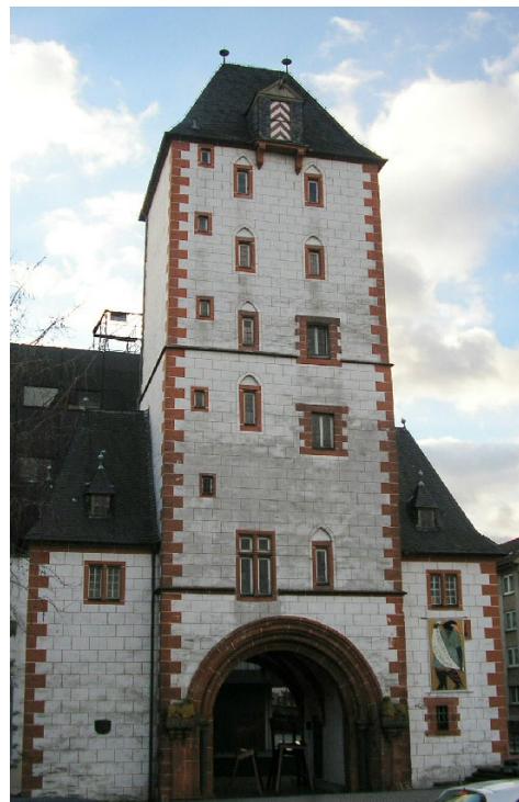
Tower in Eisenturm
