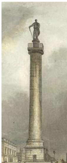
Original design of the column with the Emperor's statue atop the platform
